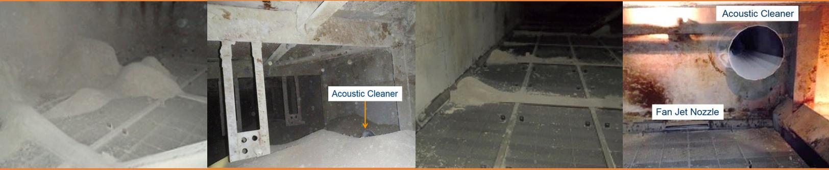
Ash buildup in coal-fired SCR reactors is a common occurrence that negatively affects gas flow and catalyst life. CORMETECH employs a combination of acoustic cleaners and ash sweepers to eliminate this industry-wide problem and offers the following features:
